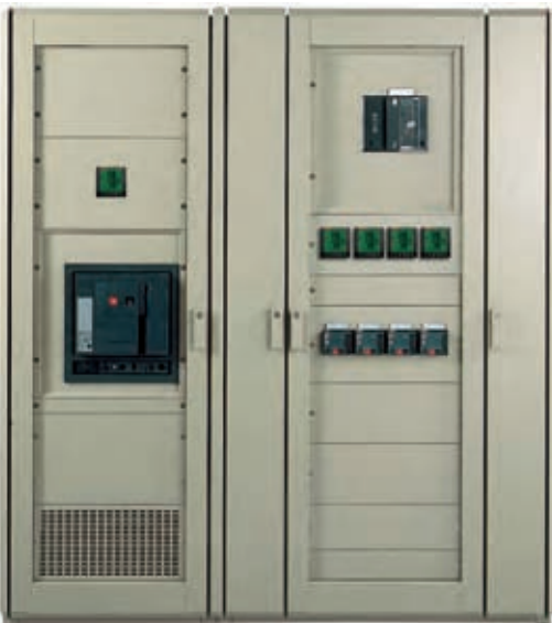
Main LV switchboard.
