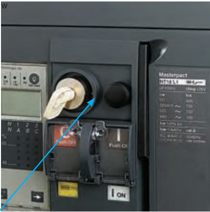
Electrical closing pushbutton BPFE.
